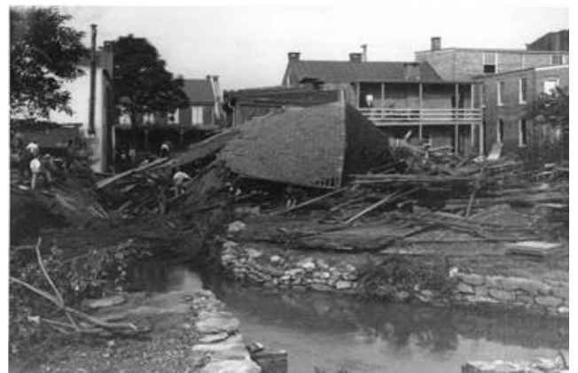
Mill Creek flood debris, South 3 rd Street
