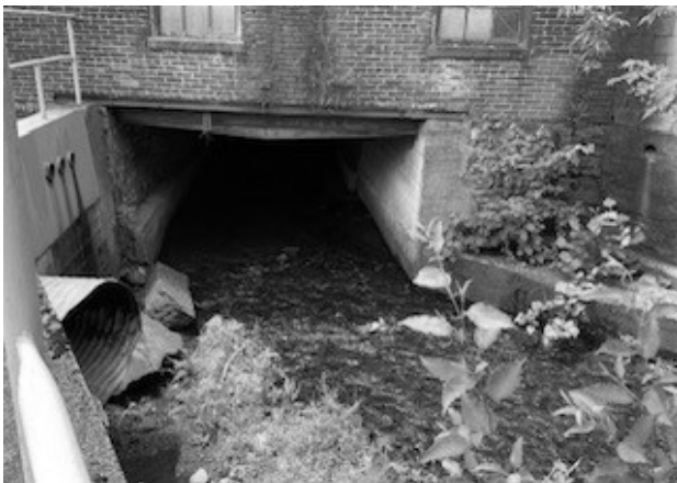
Kaercher Creek drops under Plow Works at 4 th Street
