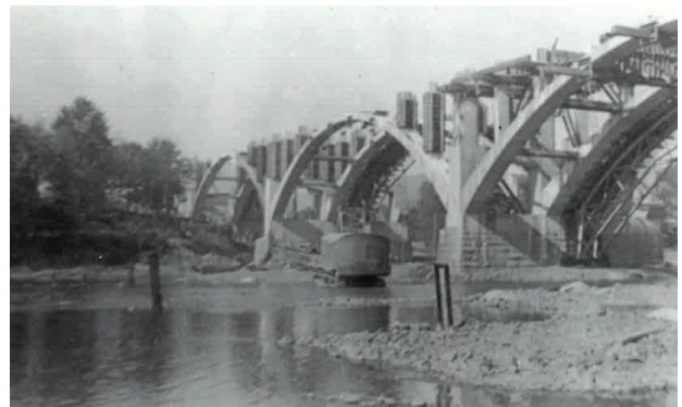
Route 122 bridges under construction, early 1950s
